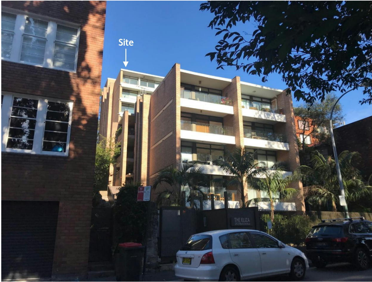
view of site from Billyard Avenue
